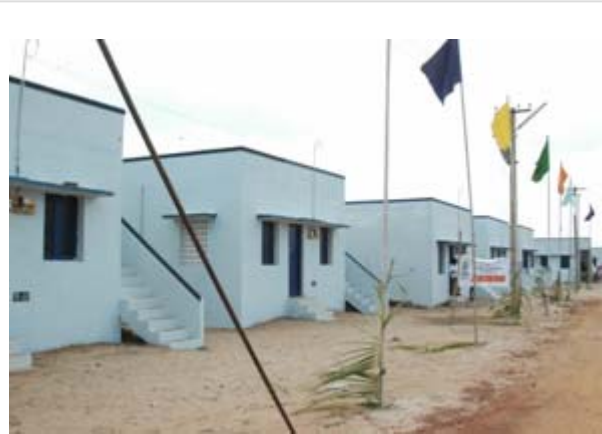
50 Houses Constructed by Guru Nanak Sarbat Sikh Sangat for Tsunami Affected people at Muzhukkuthurai village in Killai Taluka, Cuddalore District, Tamil Nadu, India.
